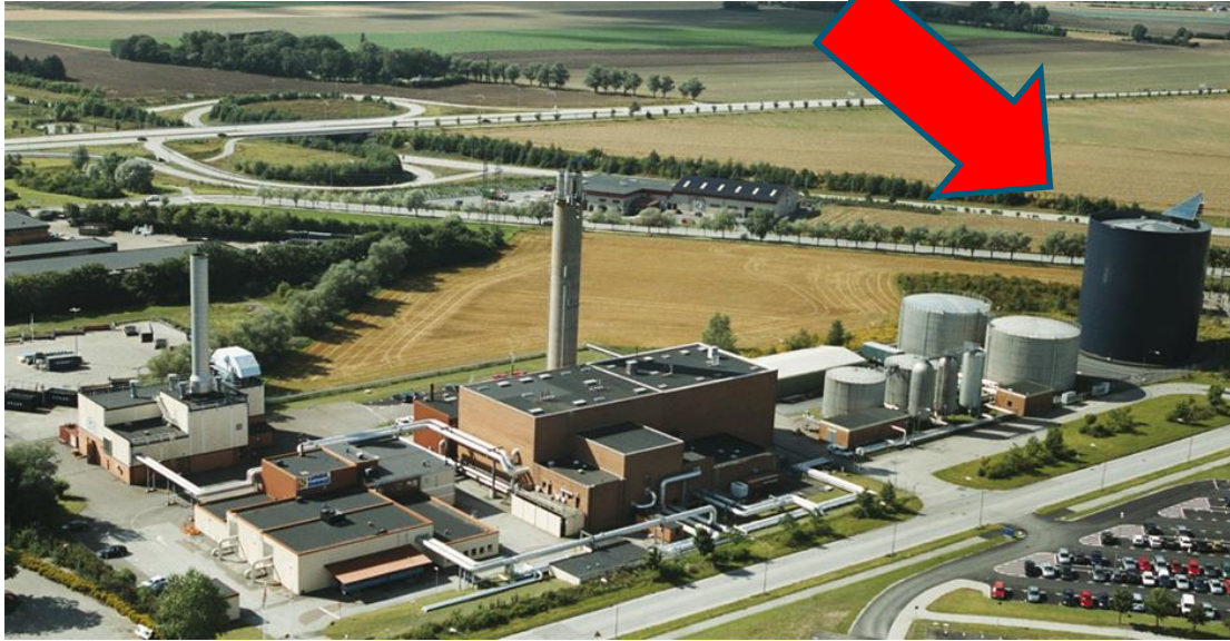
Hot water storage for district heating, Gunnesbo
